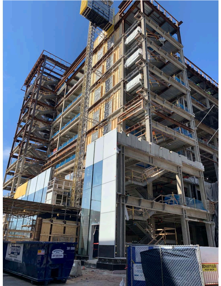
Installation of glass on the tower floors of the McGivney Tower.
